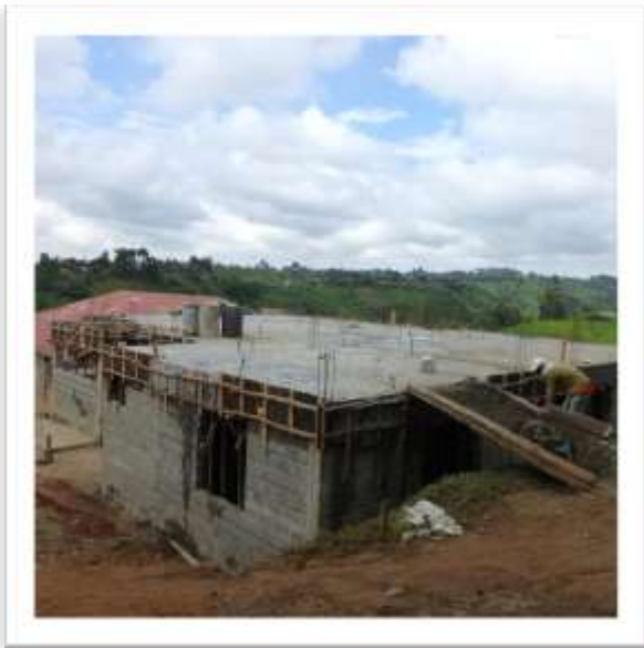
Front side of ground floor building
