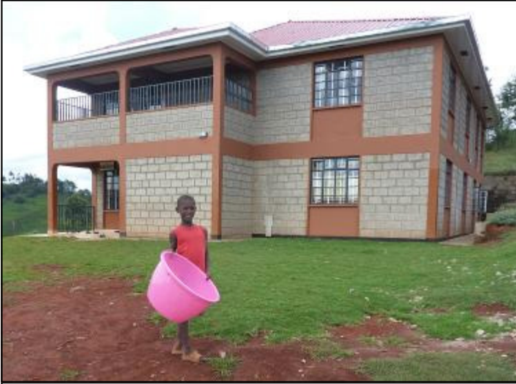
The top floor has been completed and is ready for a new family!
