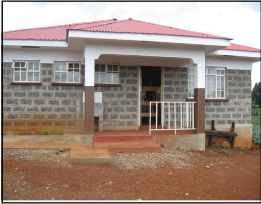
Bunkhouse, complete with toilet and shower, for ministry teams to stay!
