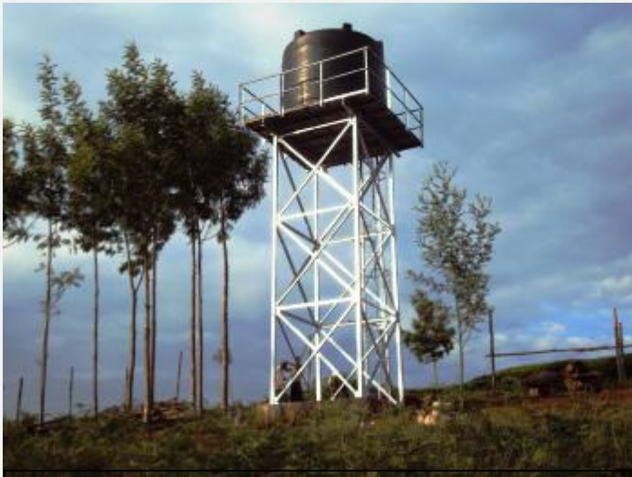
Elevated water tower. Just a little more painting to be done.
