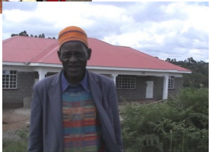
This man is clearing the land and planting beautiful bushes around the fence lines that will help keep out intruders. The finished building is behind him.
