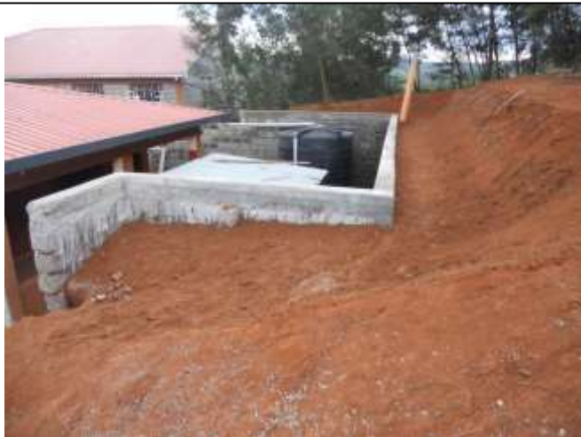
The completed retaining wall behind the kitchen.
