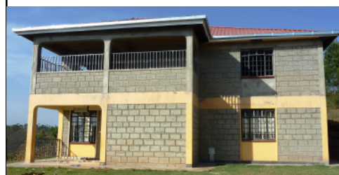
Work continues on the top floor
