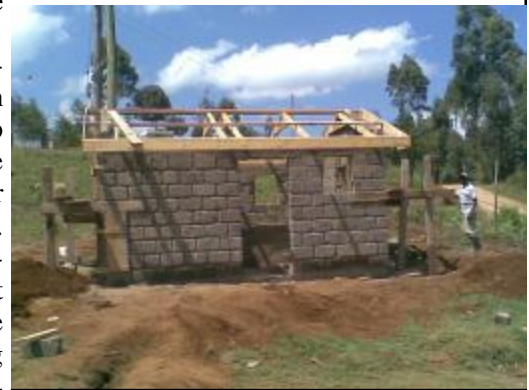
The pump/electric/guard house under construction
